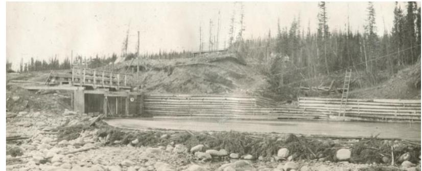
c. 1909-13: North Fork Penstock intake under construction. The Gatehouse has not yet been installed on top of the pressure boxes and penstocks (Yukon Archives).
