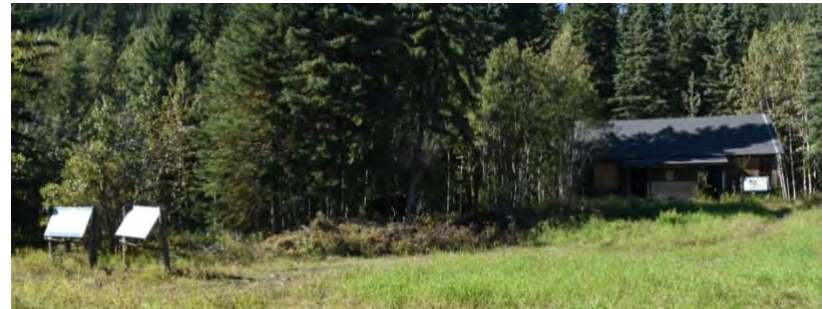
2021: Looking west at the Telegraph Office and interpretive signage (Historic Sites Unit, Yukon).
