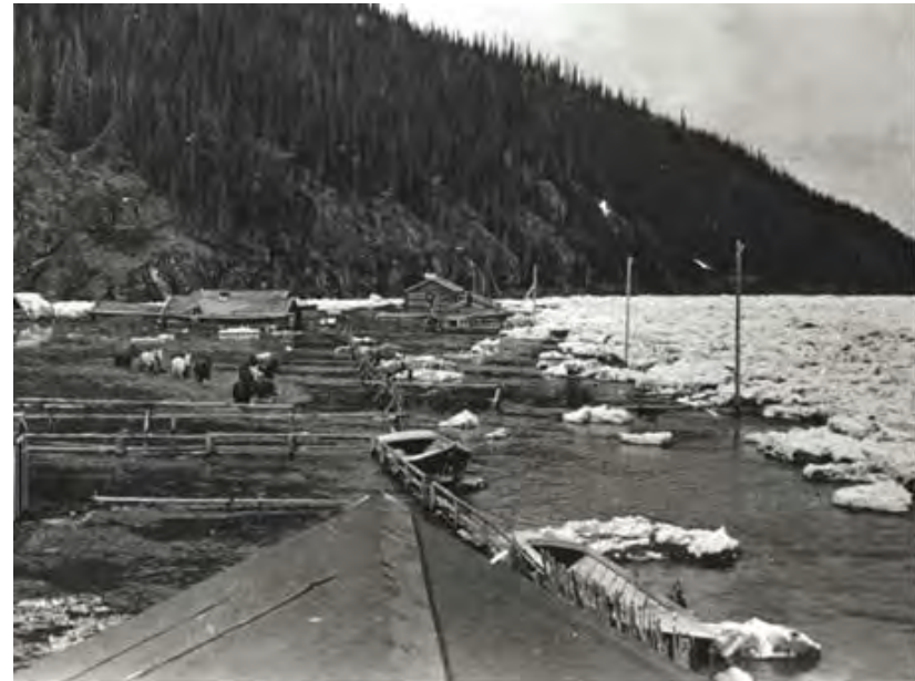
Undated: Yukon Crossing settlement looking west during a spring floor (Yukon Archives).
