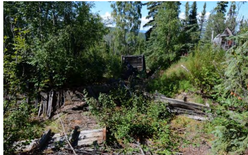
2015: Decaying Trail Gulch infrastructure components (Historic Sites Unit, Yukon).
