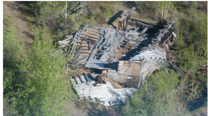
2004: Aerial view of collapsed Gatehouse (Historic Sites Unit, Yukon)
