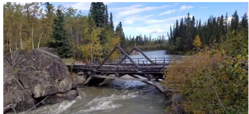
2020: Looking north to Canyon Creek Bridge (Historic Sites Unit, Yukon).
