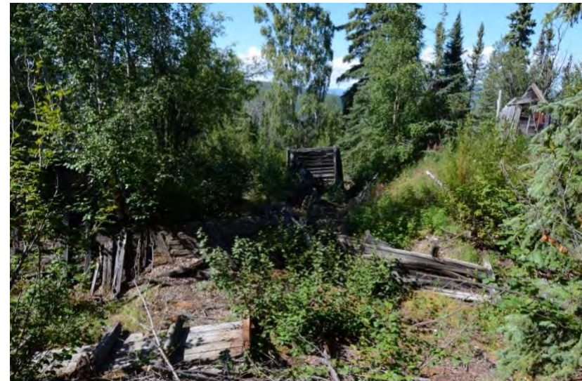
Collapsed infrastructure at the Trail Gulch Heritage Reserve (HSU).
