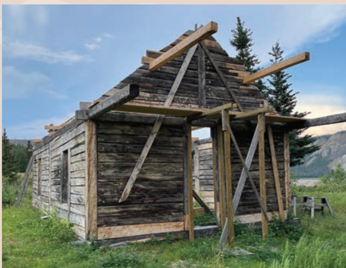
St. Luke's Anglican Church conservation. Rampart House. 2023
