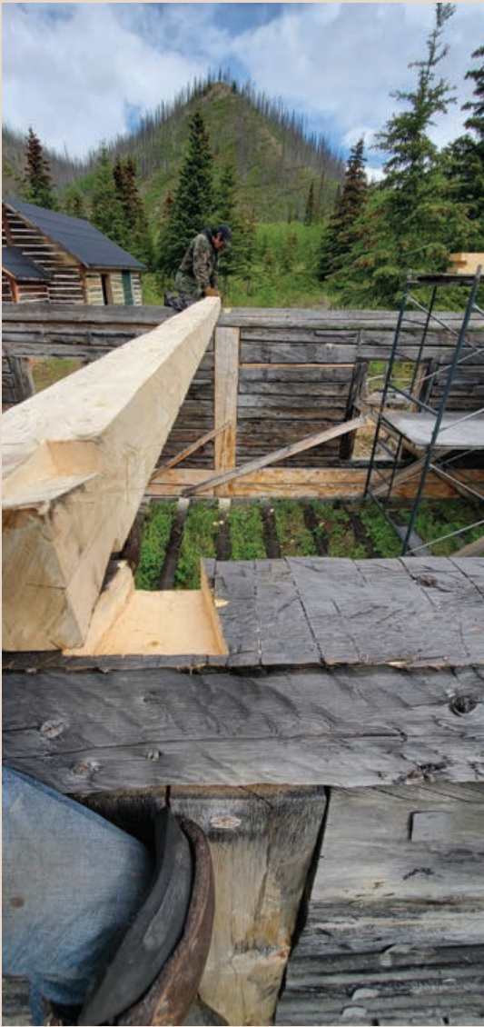
Cross piece ready to install. Rampart House Church. 2023.
