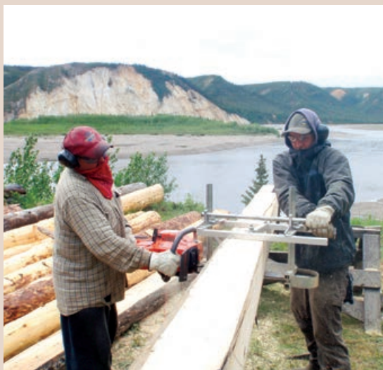
Harvey Kassi and Donovan Frost, west side job site. Rampart House. 2016.
