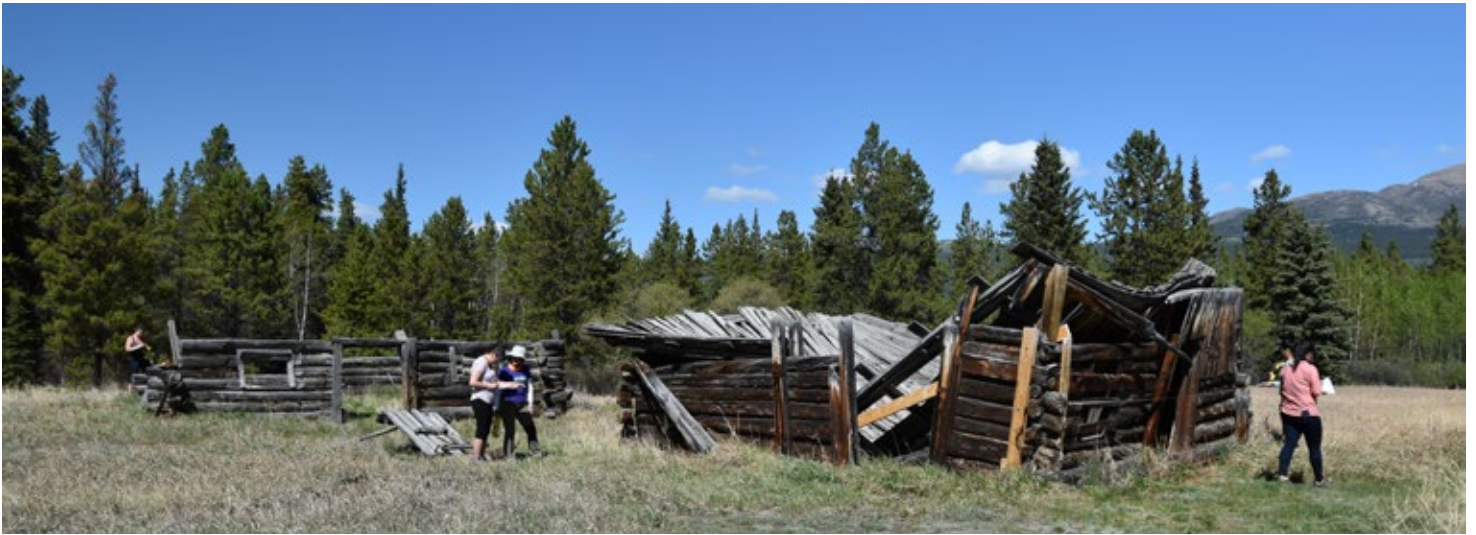
Students take measurements of buildings at Robinson Roadhouse during the 2019 Yukon College Heritage and Culture Field School.
