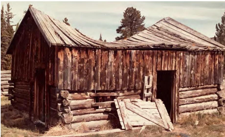
Photo credit: John Schwindt. Robinson area building circa 1978.
