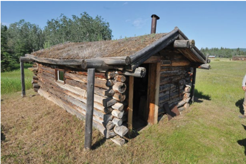
▲ The Tommy McGinty Cabin before work began. June 2024
