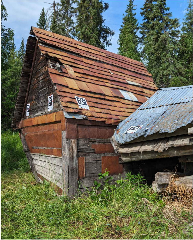
SOUTH ELEV. PARTIALLY OBSTRUCTED 8 CURRENT CONDITION (2024) AH107
