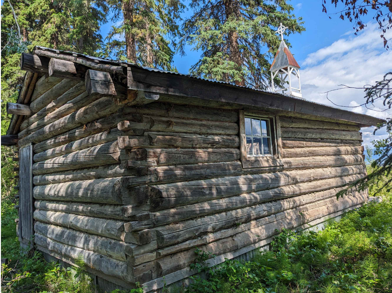
SOUTH-WEST ELEVATION 8 CURRENT CONDITION (2024) AH106
