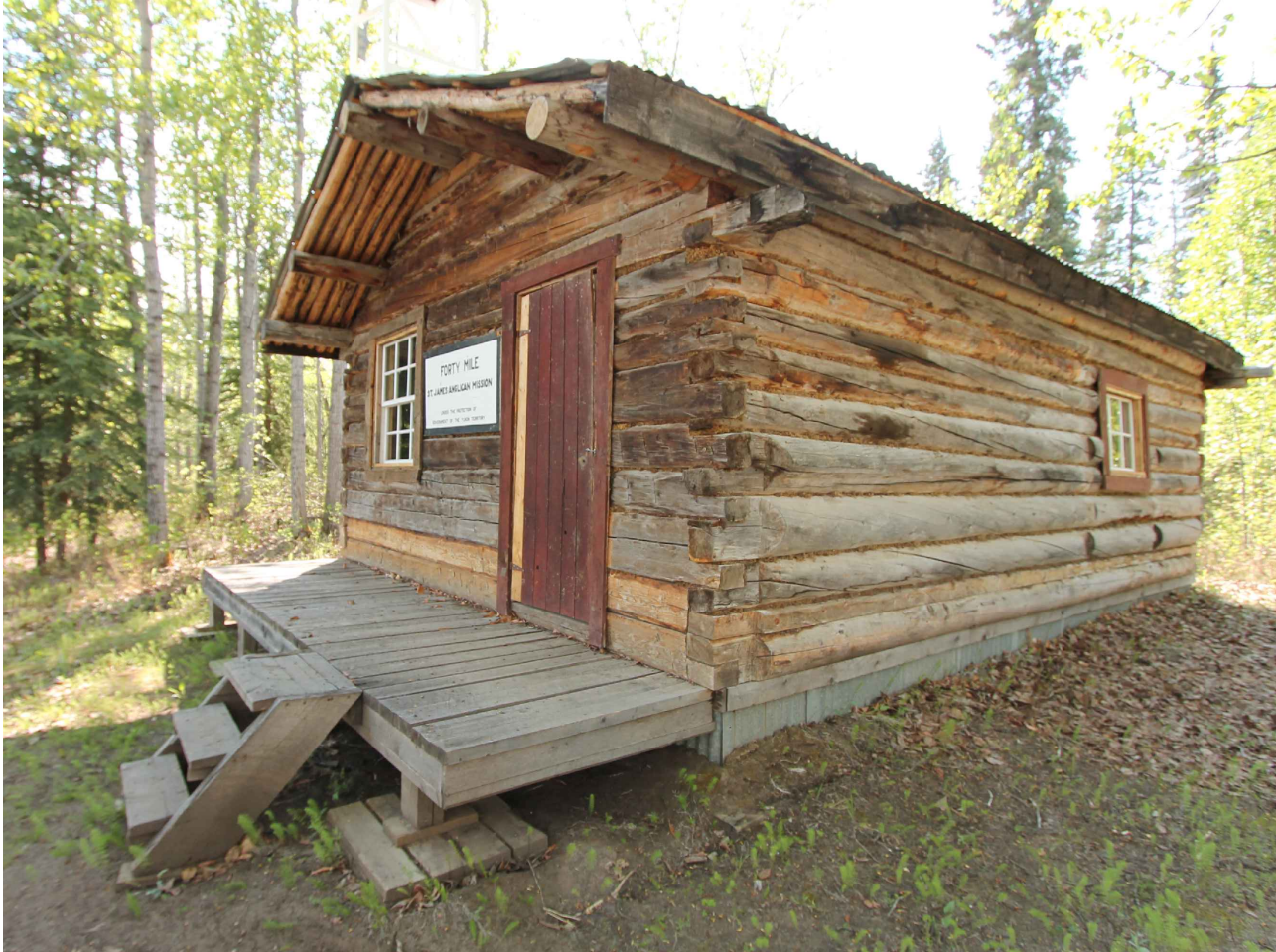
NORTH-EAST ELEVATION 6 PREVIOUS CONDITION (2015) AH106
