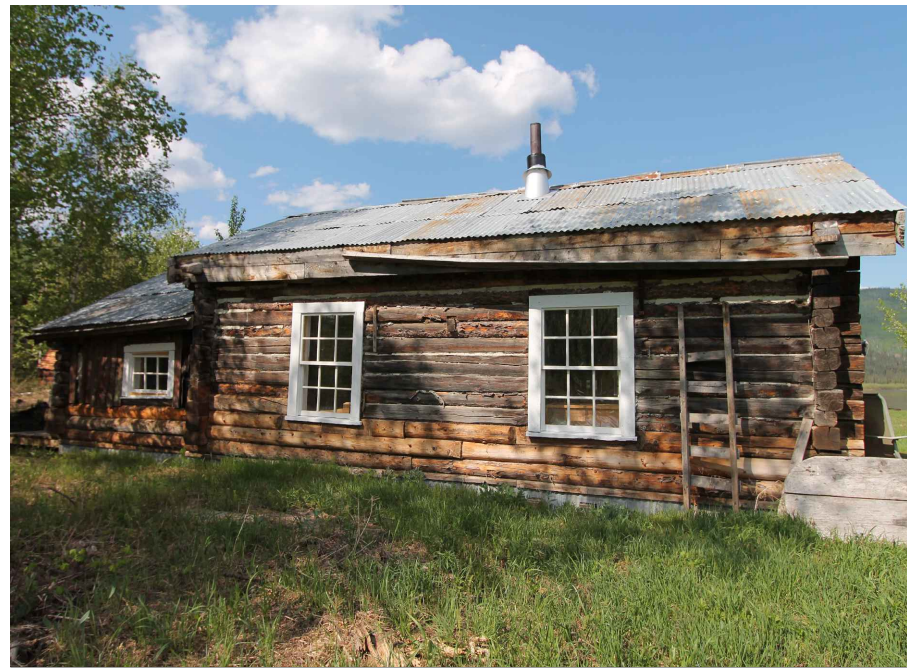
EAST ELEVATION 10 PREVIOUS CONDITION (2015) AH102
