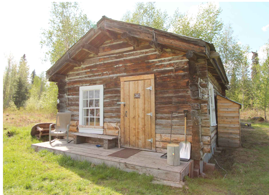
WEST ELEVATION 6 PREVIOUS CONDITION (2015) AH102
