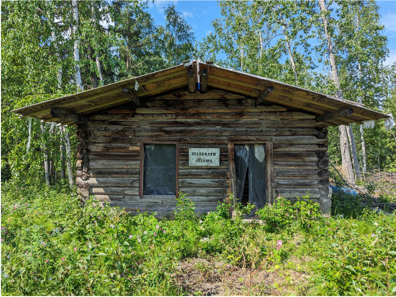
EAST ELEVATION CURRENT CONDITION (2024) AH103
