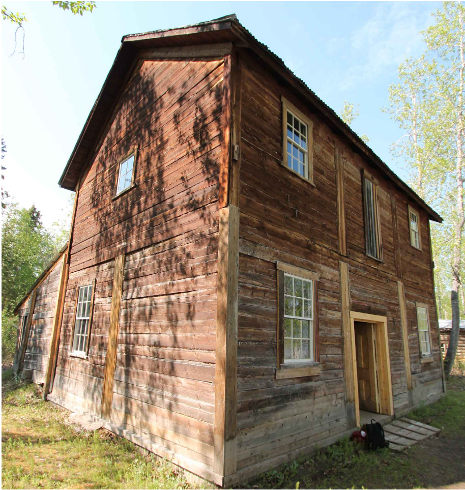
SOUTH-EAST ELEVATION PREVIOUS CONDITION (2015)
