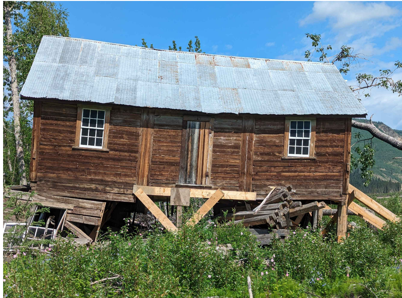
EAST ELEVATION CURRENT CONDITION (2024)
