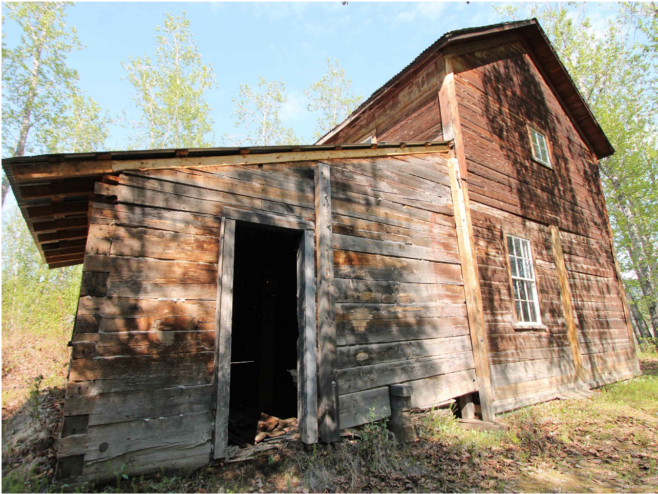
SOUTH ELEVATION PREVIOUS CONDITION (2015)
