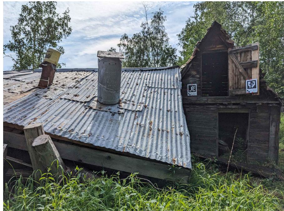
REMAINING ROOF STRUCTURE 7 CURRENT CONDITION (2024) AH102
