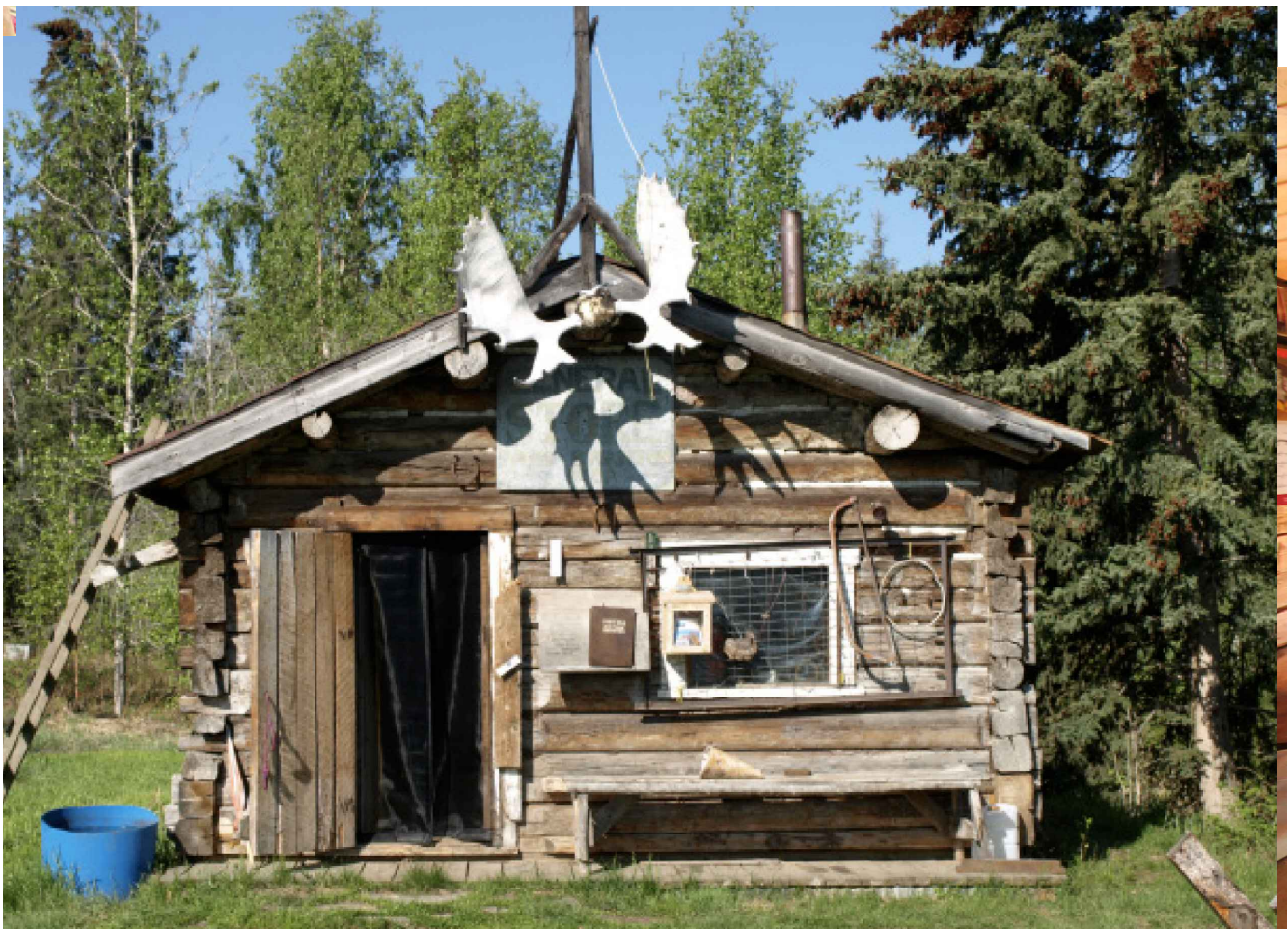
EAST ELEVATION PREVIOUS CONDITION (2015) AH101
