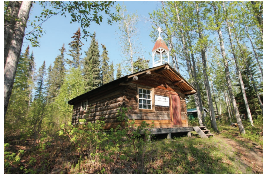
BEFORE: Anglican Church (ERA, 2015)
