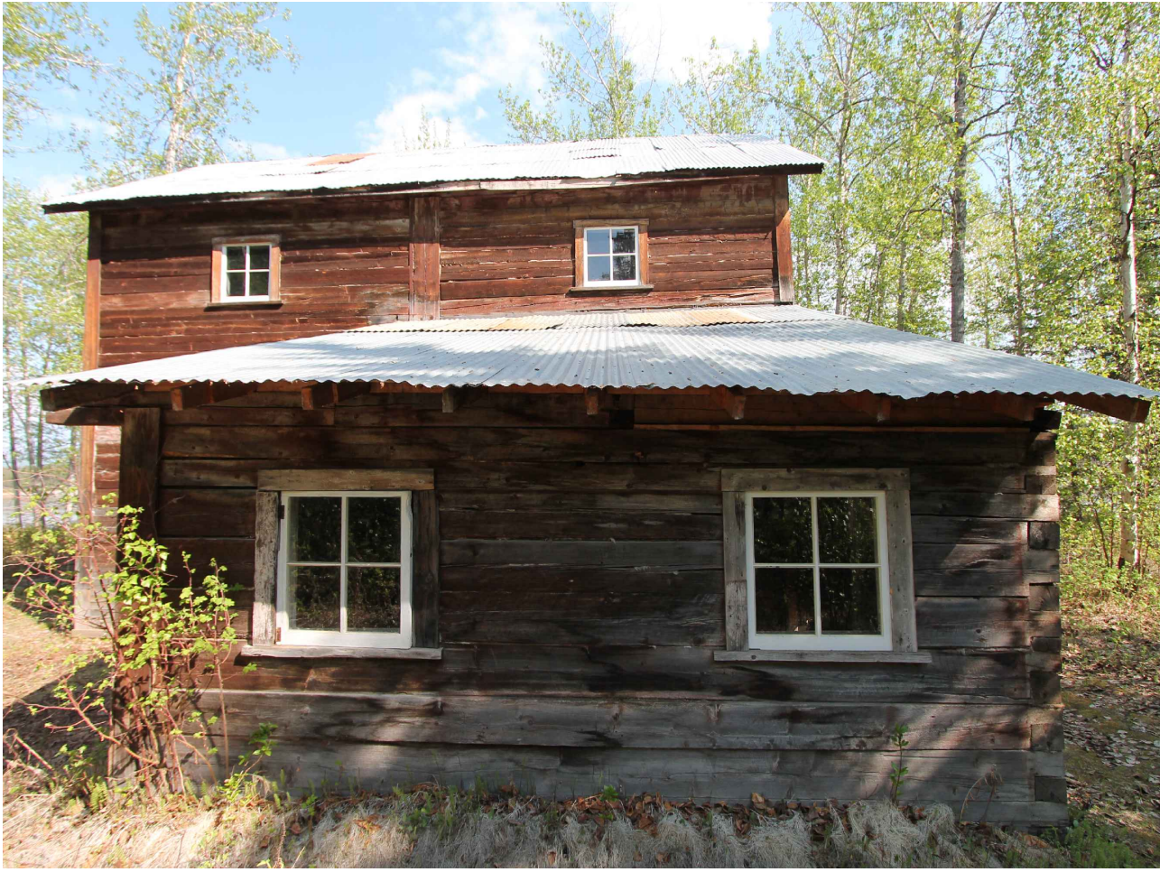
WEST ELEVATION PREVIOUS CONDITION (2015)
