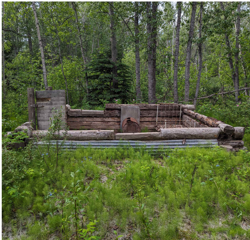
REMAINING STRUCTURE CURRENT CONDITION (2024) AH108
