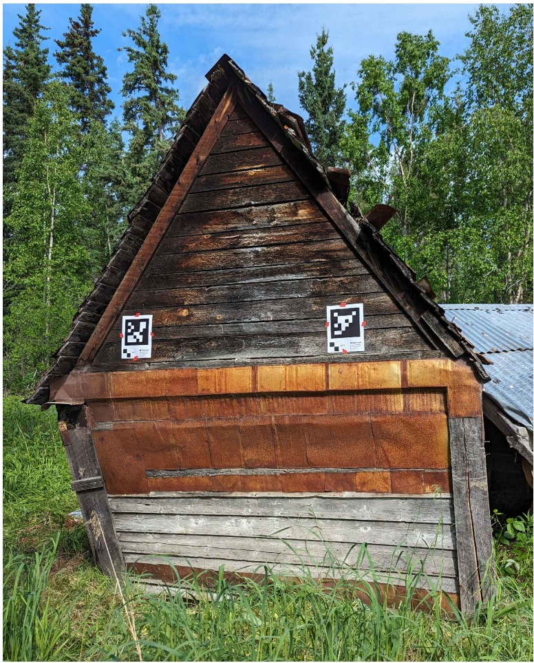
WEST ELEVATION 7 CURRENT CONDITION (2024) AH107
