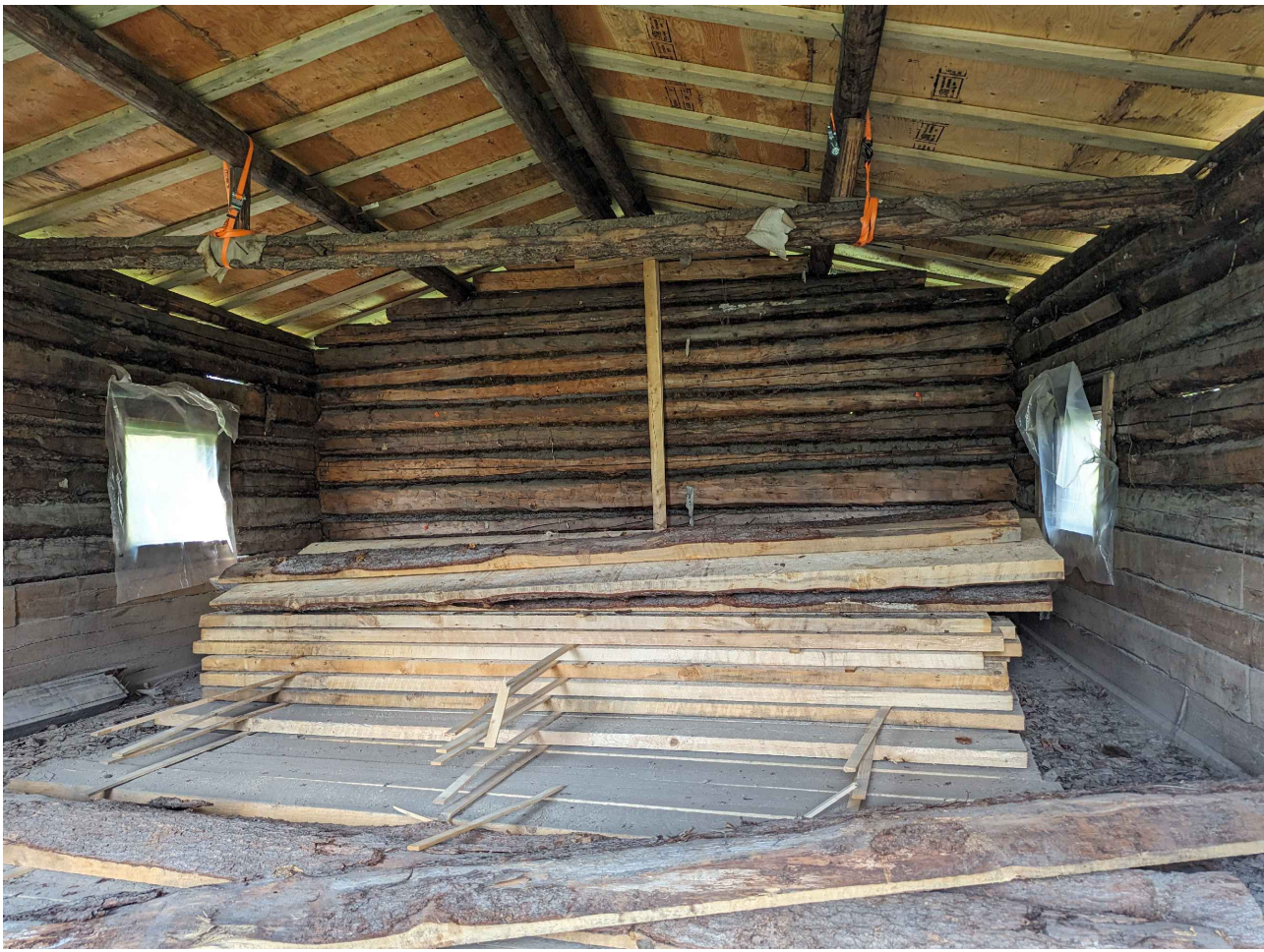
INTERIOR CURRENT CONDITION (2024) AH103
