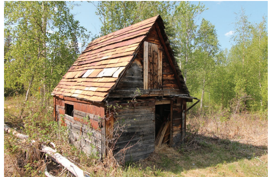
BEFORE: Metalworking Shop (ERA, 2015)
