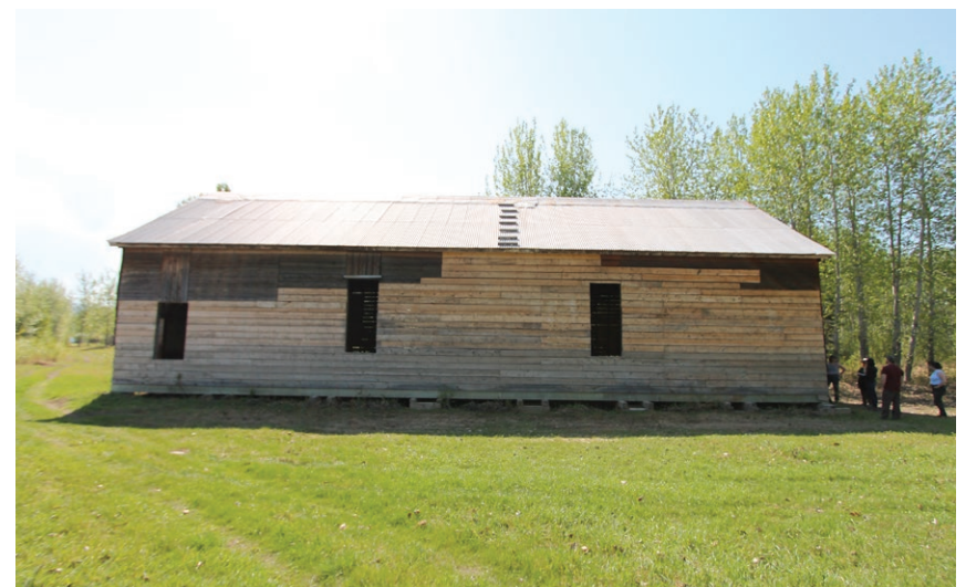
BEFORE: Alaska Commercial Company Warehouse (ERA, 2015)
