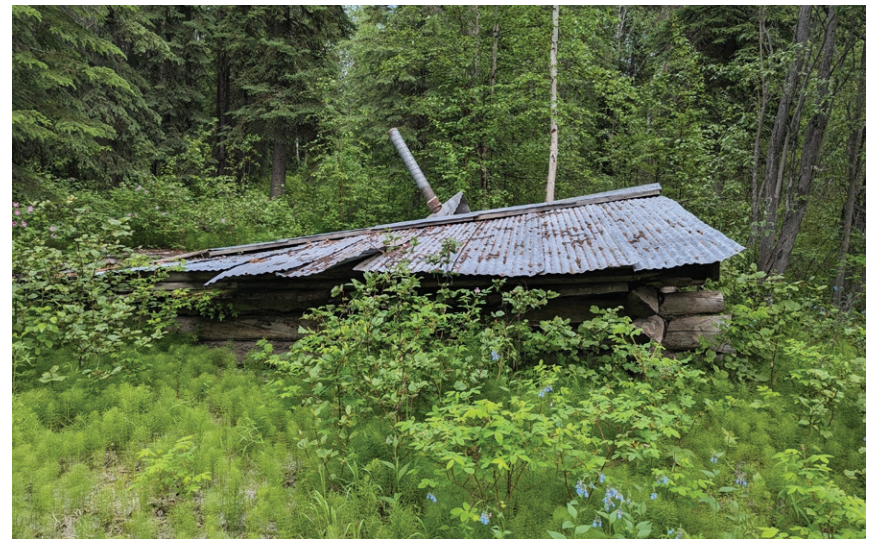
AFTER: Willie DeWolfe Cabin, base above and top half below (ERA, 2024)
