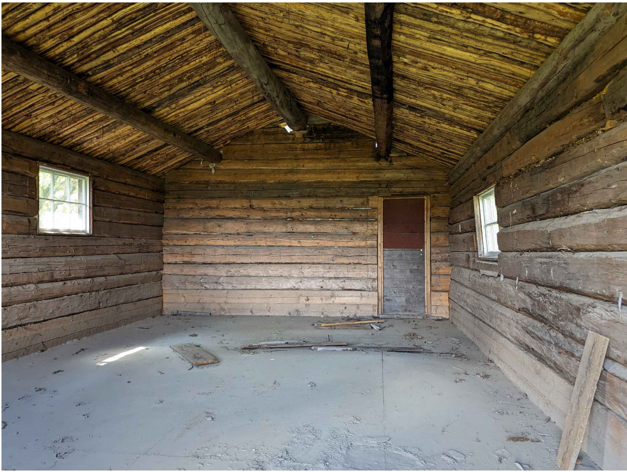
INTERIOR 9 CURRENT CONDITION (2024) AH106
