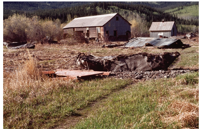
1979 flood and ice-jam aftermath, showing building destruction near the confluence of the two rivers (YG).
