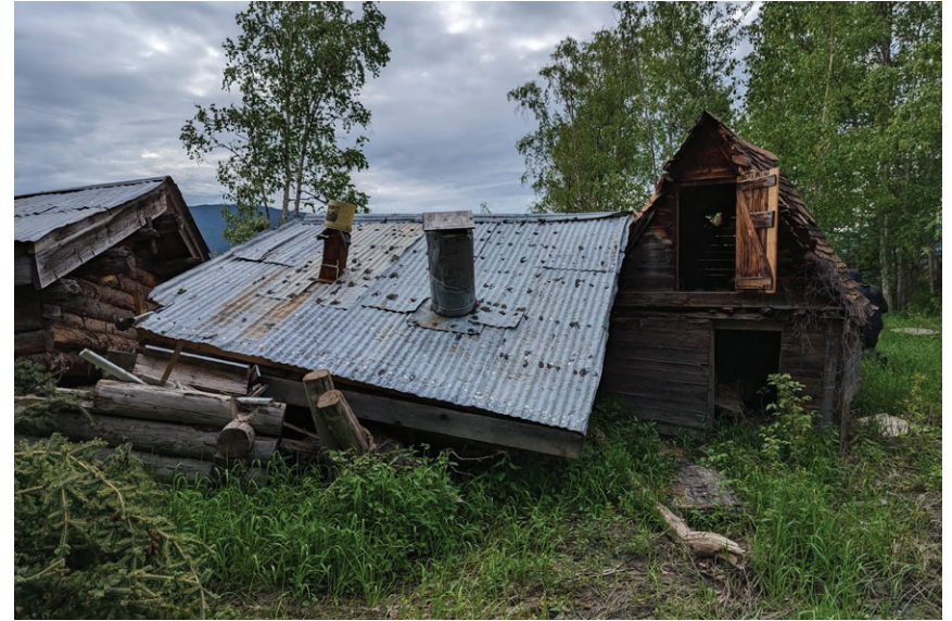
AFTER: Metalworking Shop (ERA, 2024)
