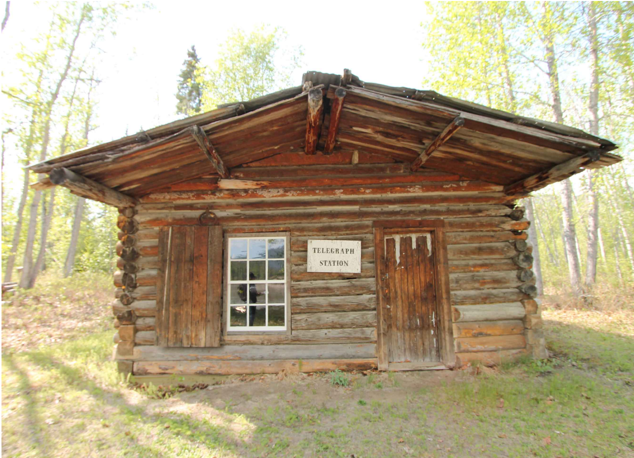
EAST ELEVATION PREVIOUS CONDITION (2015) AH103
