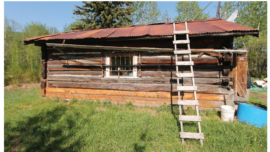
BEFORE: Swanson's Store, side elevation (ERA, 2015).
