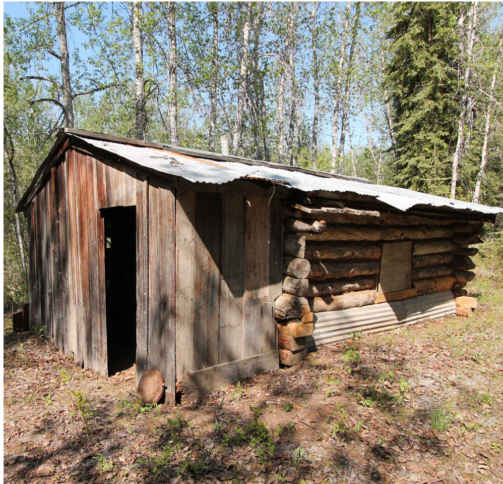
NORTH-EAST ELEVATION PREVIOUS CONDITION (2015) AH108
