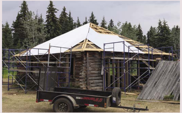
▲ Cladding the roof after structural stabilization.
